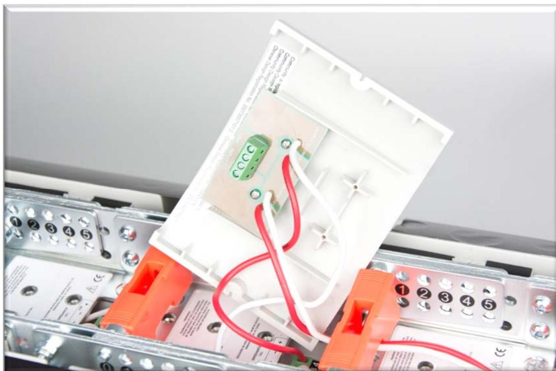
Fit the HAM03191 flying bracket (arrowed) to the top O-Line™ module of the array.
