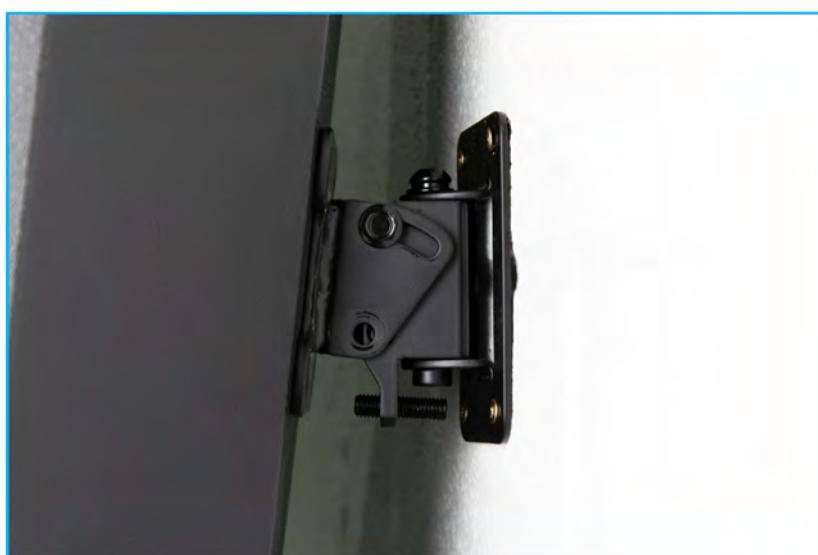
Once the bracket is hooked together and taking the weight of the cabinet you can replace the lower bolt.
