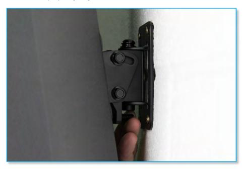
Once the vertical position is fixed the two horizontal bolts can be tightened, this is best achieved by using a socket set with an extender bar to reach the bolt heads.
